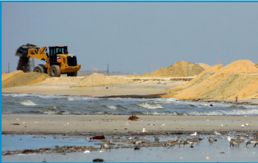
Kimbles Beach during 2014 restoration
