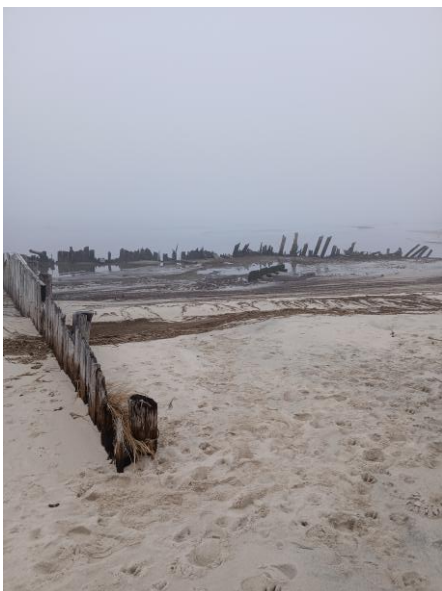
Triangular derelict bulkhead (rubble).
