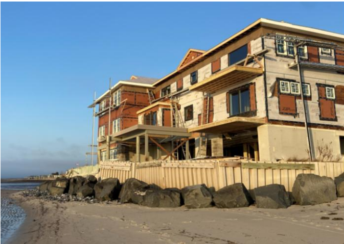
Bin blocks/riprap surrounding house .
